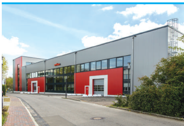
The new Staple Fiber Technology Center in Neumünster - with around 2,100 m 2 one of the largest in the world.
